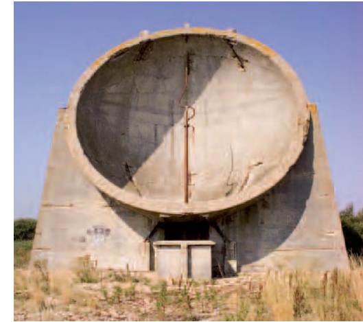
Fig 71 Top, one half of a stereo pair taken for the photogrammetric survey of the acoustic mirror array at Greatstone-on-Sea: the microphone site can be seen clearly; upper-middle, the wire frame derived from the stereo pairs presented in CAD; lower-middle, the point cloud data from the laser scanning – the post spacing was 10mm and the colours indicate variation in the reflectance of the surfaces recorded; bottom, rendered scene of the textured model derived from the laser scan point cloud and the site imagery. The model incorporated edge data from photogrammetry.
