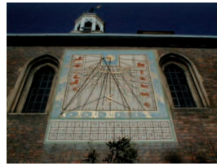
Fig 10 Rectified photography of a sundial: the severe camera tilt has caused scale variation, which is removed by rectification. Once rectified, the image can be used for scale drawing, provided the tracing is only on the plane of rectification.
