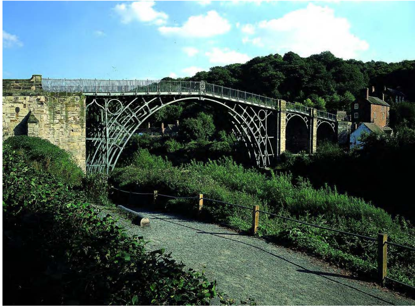
Fig 52 The Iron Bridge at Coalbrookdale. This was the world's first major iron-span bridge, erected in 1779 under the direction of Abraham Darby III (1750–91).
