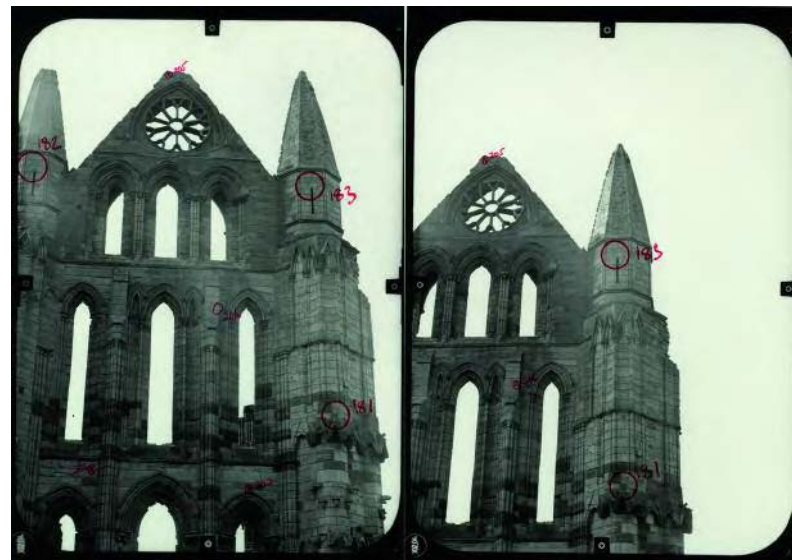
Fig 13 Stereo pair of Whitby Abbey: eight stereo pairs were required to provide complete cover of the north face of the North Transept of Whitby Abbey church. The metric camera used for this pair was of 5in x 7in format with a 300mm lens. The red notation on the stereo pair marks the targets and detail points used for control. Note the fiducial marks on the border of the image: here they take the form of small circles, although the type of mark depends on the camera.
