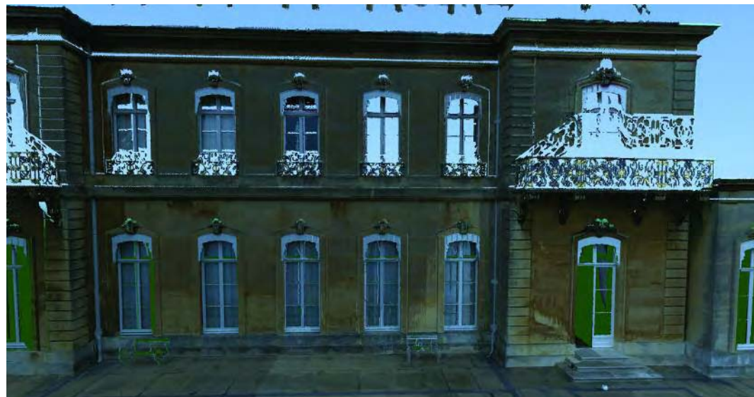
Fig 22 Phase based scanner data with RGB overlay: this image of a 3-D data set shows the coverage possible from a terrestrial scanner. The patches of 'sky' in the facade are areas where there is no data due to interference from obstructions, in this case the cornice and balcony railings. The simultaneous capture of RGB data adds to the richness of the model.
