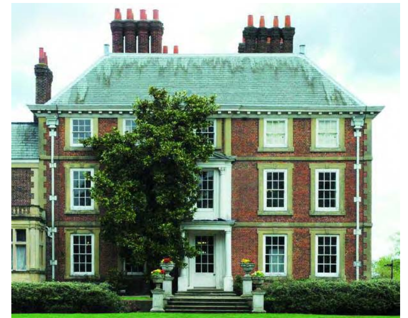
Fig 32 Without reconnaissance this facade might have been surveyed using an inappropriate technique due to a lack of provision for either infill survey behind the tree or clearance of the facade. A reconnaissance visit will repay the time spent many times over in cases like this.
