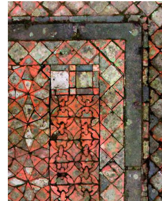
Fig 8 Image-based methods are good for the capture of texture and colour. This medieval tiled floor detail is recorded, complete with its condition; wear and accretion are clearly visible in this rectified photomosaic prepared for 1:20 reproduction.
